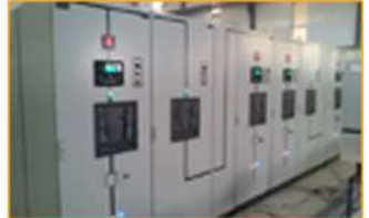
Testing & Commissioning of Substation- Up to 765kV
